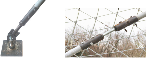
Figure 10: Connections devised jointly by the Navier laboratory and the company T/E/S/S. Left: Pin anchorage for beams. Right: Assembly used to join two beams.
