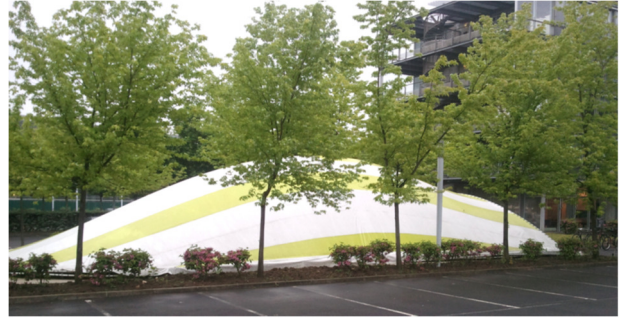
Figure 5: Long term erected composite gridshell. Some planar parts (yellow) of the membrane can be seen.
