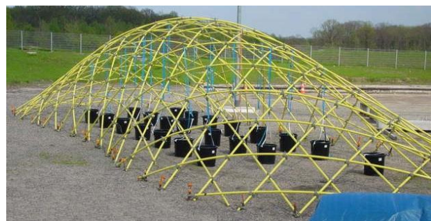
Figure 6: First experimental gridshell under testing.
