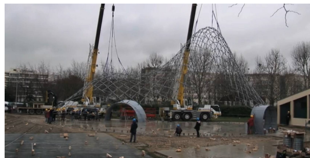
Figure 2: Cathedrale Ephemere de Creteil. Primary grid deformed elastically and about to be attached to boundary conditions.
