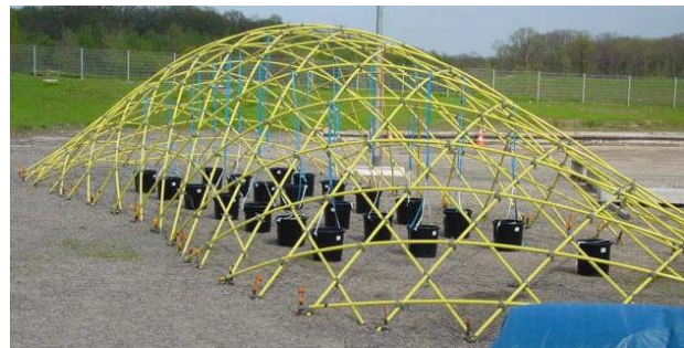
Figure 6: First experimental gridshell under testing.
