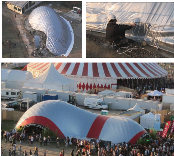
Figure 9: Up: Positioning of the PVC coated membrane (Creteil). Down: Membrane without wrinkle (Solidays gridshell).
