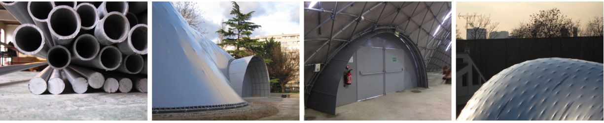
Figure. 2. GFRP tubes, steel door, grid, PVC coated fabric
