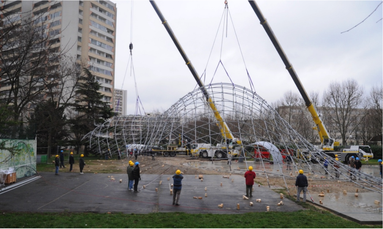
Figure. 5. Erection of the primary grid by two cranes
