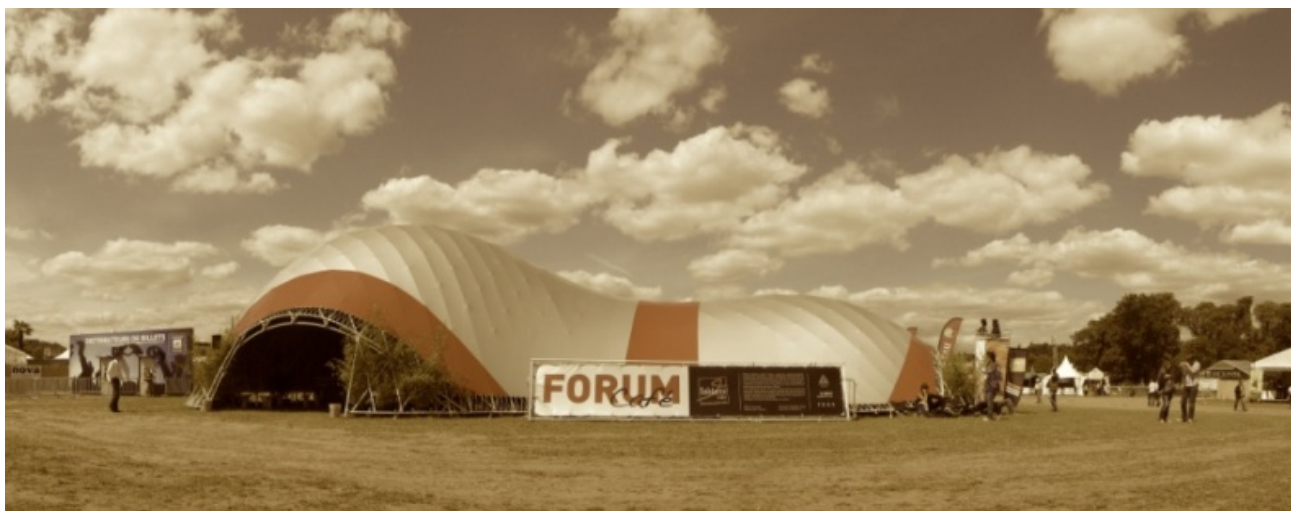
Figure 7: Photo of the final structure ( http://vimeo.com/31341461 ).
