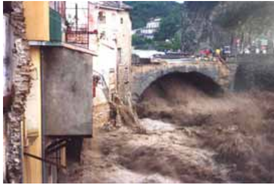
Figure 29. Flash flood in Vaison-la-Romaine on 22 September 1992. This Roman bridge, built in the 1st century AD, over the Ouvèze River resisted the flood while newer bridges and buildings collapsed. Photo by M.J. Tricart
