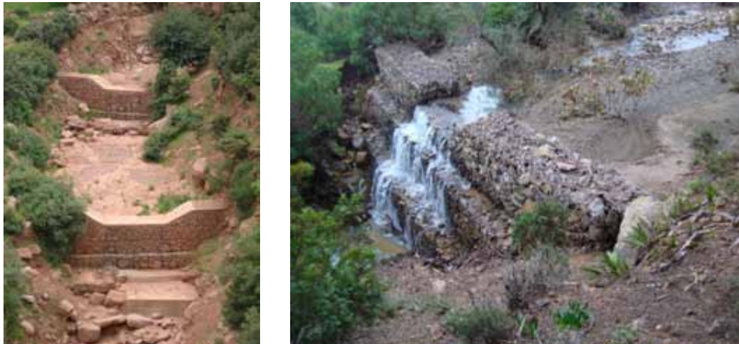
Figure 58. Torrent control equipments in Morocco. Photos by Mohamed Sabir.
