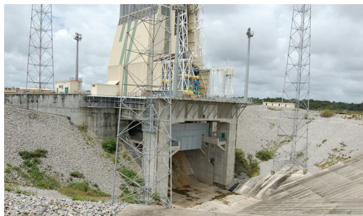
Figure 16 – Cross section geometry of the pylon installation on the Soyuz LPS and picture of the flue (flame exhaust)
