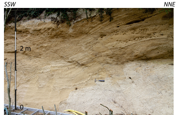
Photo 7: Major reverse fault associated with liquefaction (see also Fig. 5).
