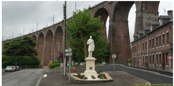
Figure 16: Statue of railway engineer Lock in Barentin (FR), the possibility of an aesthetic break (photo René & Peter van der Krogt 2012 http://www.vanderkrogt.net )
