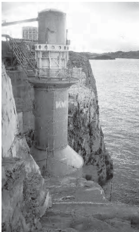
Figure 11.12. Kvaerner column in Norway [FAL 93]
