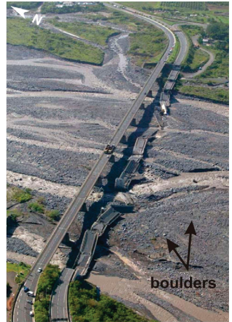
Figure 3. Photo of Rivière Saint-Etienne after Hurricane Gamède (2007). Note size of boulders (cars for scale).
