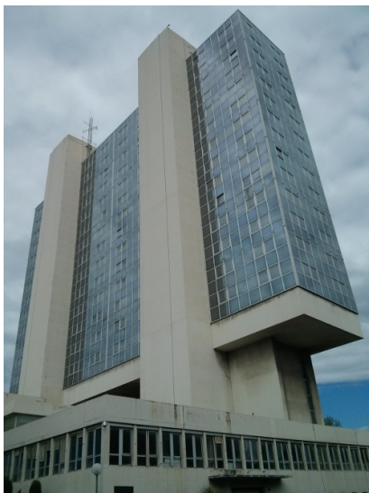
Figure 1: Side view of the building
