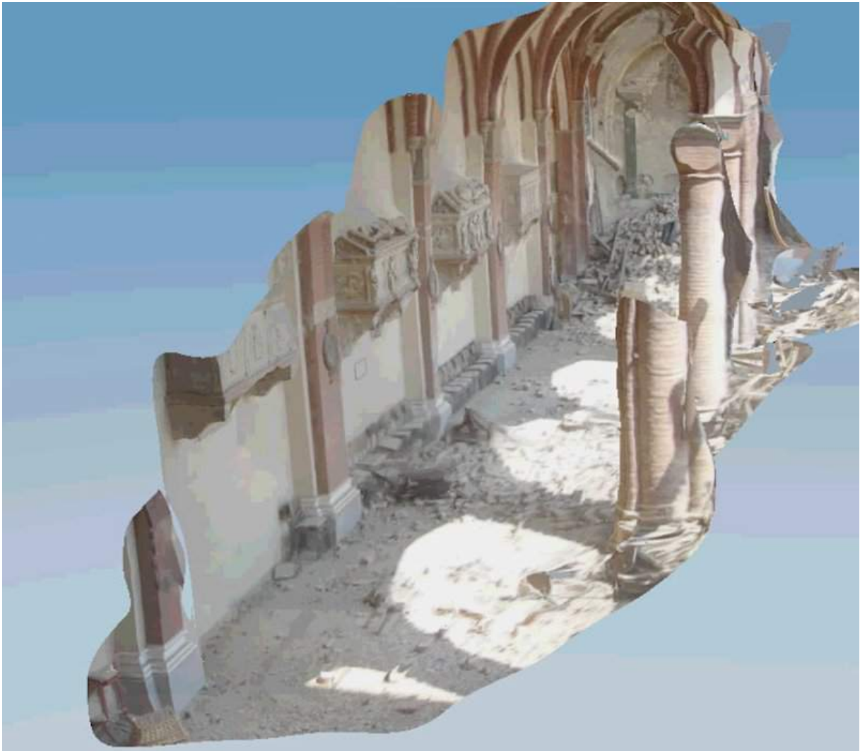
Figure 22. 3D reconstruction based on NIFTi UAV data
