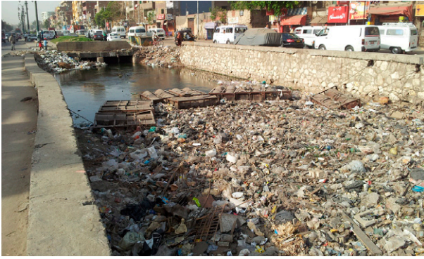
FIG. 3. The water in a channel in Giza, Egypt, is nearly completely covered by garbage and pollution. Under normal conditions, floating barrels hold back the waste, but when the flood comes, the garbage obstructs flow under bridges (in the background) and the water backs up into neighborhoods. Such micro-scale behavior is difficult to monitor, let alone to model or predict.
