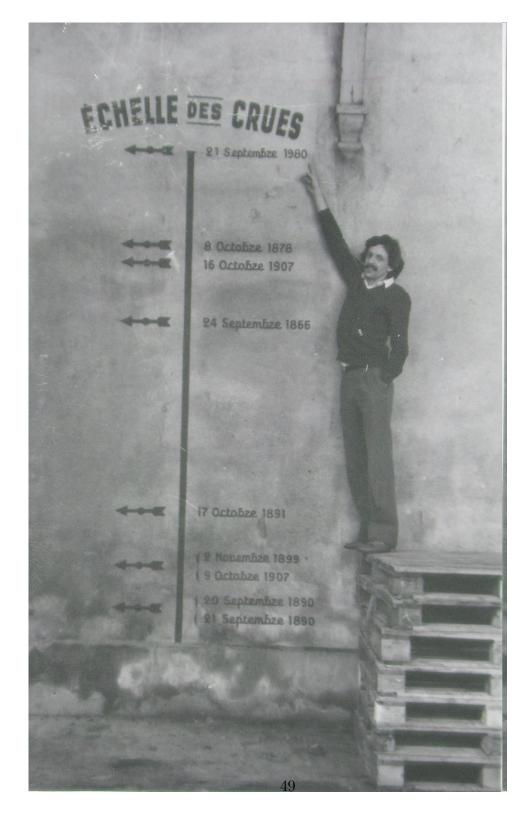
Figure 1: Flood marks on the Loire river at Puy-en-Velay (France).
