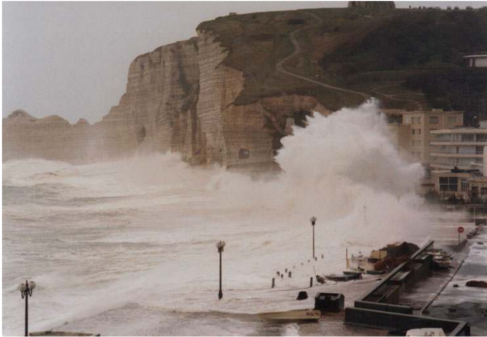
Fig. 4.6 Storm surges at Etretat in 27–28/02/1990 (Photo S. Costa)
