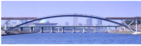
Fig. 1: Seonyu Footbridge built with RPC
