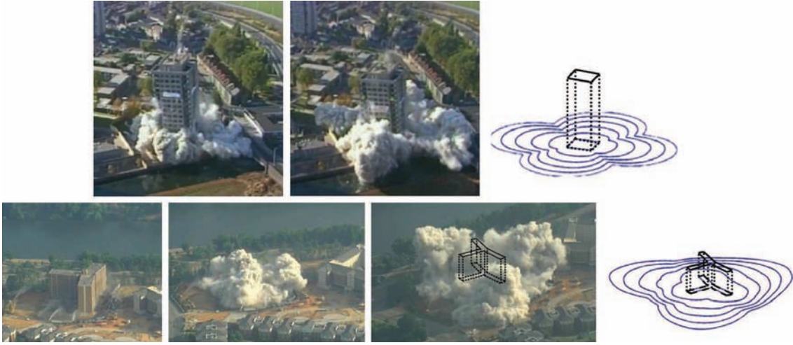
Fig. 1 Field observations of a non-circular gravity current. Aerial views of ( top ) a building of square cross section and ( bottom ) a T-shaped building being demolished. The structure of the debris cloud is highly dependent on the building's shape. Observe that material very close to the center of the building moves farther out than material located at the building's extremities. The dynamics of the cloud is reasonably well captured by our proposed model, where the front location of the cloud is marked at equal instants of time as blue lines (color figure online)
