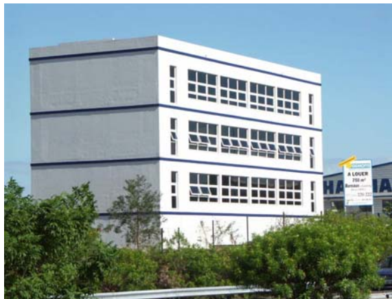
Figure 1: A perfect counter-example in thermal design for tropical climate building. The unprotected glass frontage faces east.
