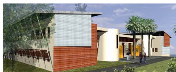
Figure 4 : View of the northerly facades (solar protection with wooden strips) and the westerly ones (sheet metal and wood cladding).
