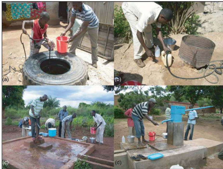
Fig. 2 Examples of the most common groundwater extraction devices and structures in the Bangui region: (a) shallow hand-dug well with a used tyre as a curb; (b) shallow hand-dug well with a corroded steel barrel as a curb; (c) borehole equipped with a foot pump and protected by a concrete slab; and (d) borehole equipped with a hand pump.
