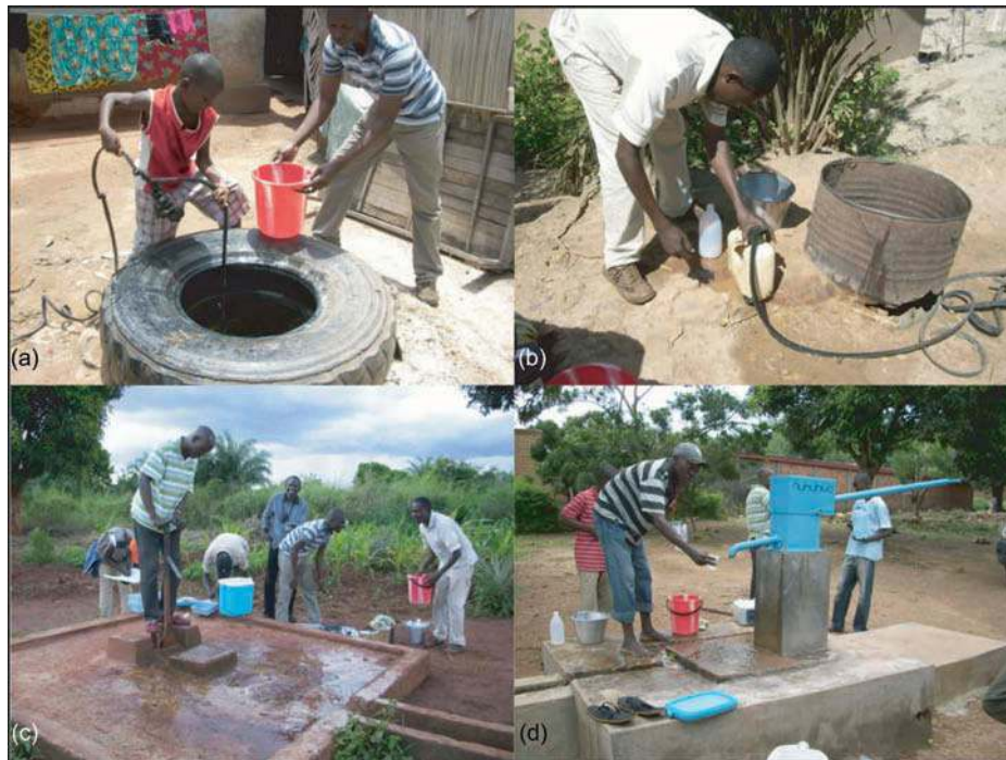
Fig. 2 Examples of the most common groundwater extraction devices and structures in the Bangui region: (a) shallow hand-dug well with a used tyre as a curb; (b) shallow hand-dug well with a corroded steel barrel as a curb; (c) borehole equipped with a foot pump and protected by a concrete slab; and (d) borehole equipped with a hand pump.
