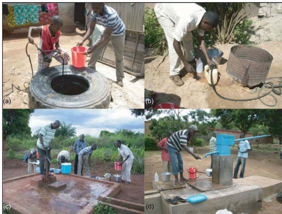
Fig. 2 Examples of the most common groundwater extraction devices and structures in the Bangui region: (a) shallow hand-dug well with a used tyre as a curb; (b) shallow hand-dug well with a corroded steel barrel as a curb; (c) borehole equipped with a foot pump and protected by a concrete slab; and (d) borehole equipped with a hand pump.
