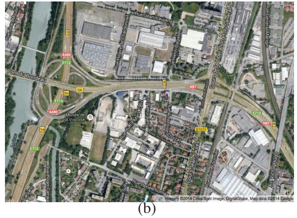
Figure 1. The south ring of Grenoble. (a) View of a stretch of the south ring, direction north-east towards Meylan (Image courtesy of DIR-CE); (b) Aerial view of the interchange “Rondeau” at the west end of the south ring (left center in the image): this site endures heavy traffic congestion during the morning and afternoon rush hours (Image courtesy of Google Maps/Satellite).
