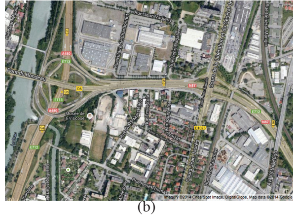
Figure 1. The south ring of Grenoble. (a) View of a stretch of the south ring, direction north-east towards Meylan (Image courtesy of DIR-CE); (b) Aerial view of the interchange “Rondeau” at the west end of the south ring (left center in the image): this site endures heavy traffic congestion during the morning and afternoon rush hours (Image courtesy of Google Maps/Satellite).
