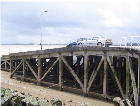
Fig.1 Blaye wharf (side view)
