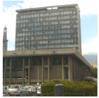
Figure 7. Grenoble city hall
