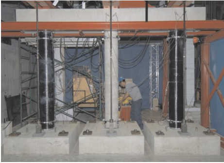
Figure 3. Bridge pier mockup with partial retrofitting.
