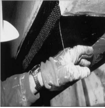
Figure 5. Beam retrofitting with FRP bonding on lower side.
