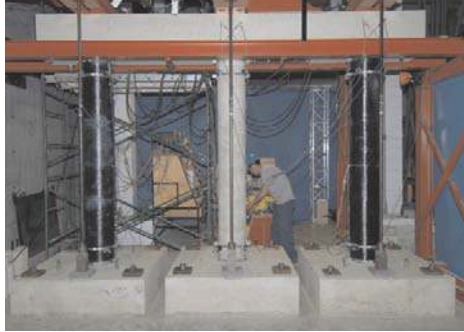
Figure 3. Bridge pier mockup with partial retrofitting.
