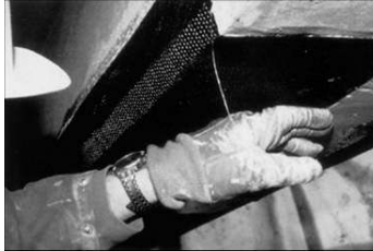
Figure 5. Beam retrofitting with FRP bonding on lower side.
