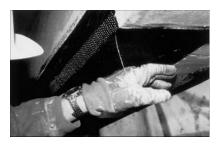
**Figure 5.1.** Increase of the flexural capacity by FRP bonding on the lower part of a beam.
