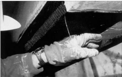
**Figure 5.1.** Increase of the flexural capacity by FRP bonding on the lower part of a beam.
