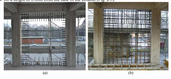
Figure 2.4. (a) Dowels and starter bars, (b) Dowels, starter bars and web reinforcement
