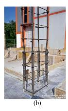
Figure 2.2. (a) Reinforcement details for beams, (b) Reinforcement details for columns
