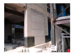
Figure 2.5. Reinforcing of the column with CFRP to safeguard against column lap-splice failure
