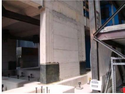
**Figure 2.5.** Reinforcing of the column with CFRP to safeguard against column lap-splice failure
