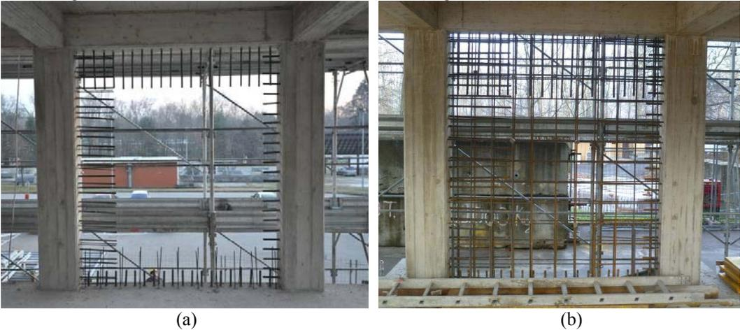
**Figure 2.4.** (a) Dowels and starter bars, (b) Dowels, starter bars and web reinforcement
