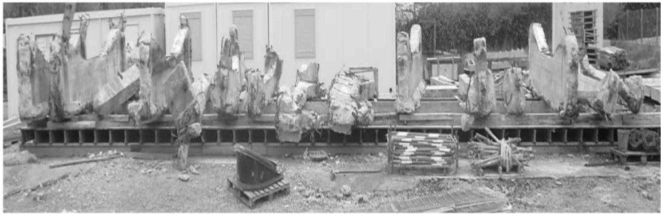
Figure 5: Beams after 80 Years of Exposure
