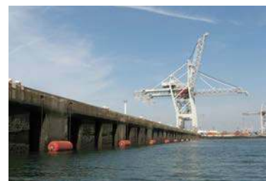
Reinforced concrete quay (Docking)
