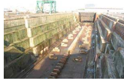
Dry dock (Construction and repair of ships)
