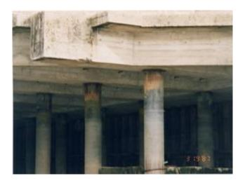
Figure 1. Steel piles with Corrosion.
