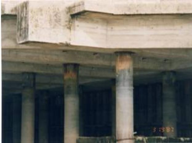
Figure 1. Steel piles with Corrosion.
