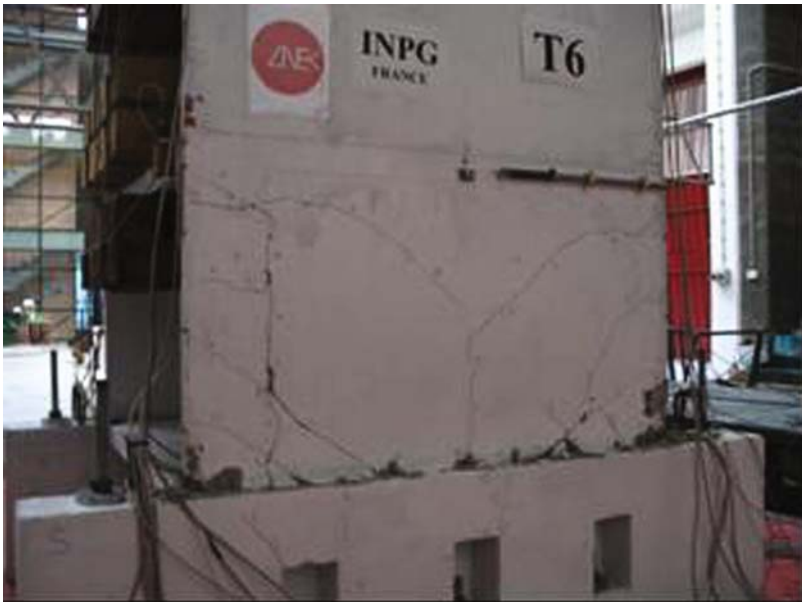
Fig. 17 Experimental damage pattern for T6 motion
