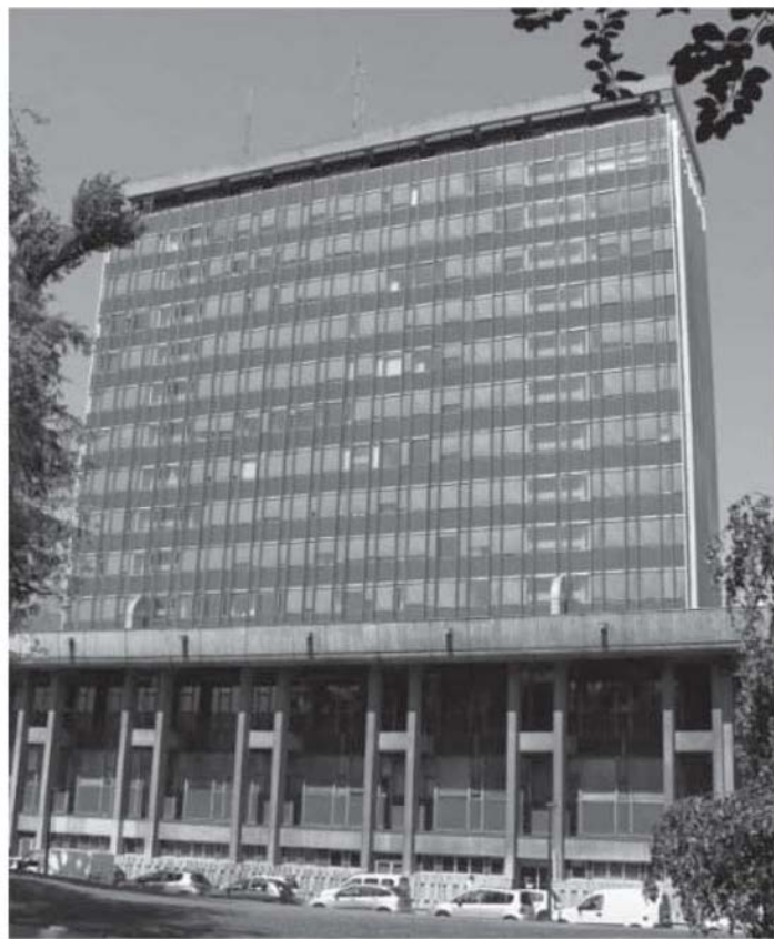
Figure 5.1. General view of the building
