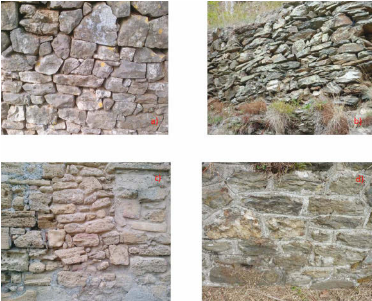
Figure 1. Irregular type of masonry a) b) d) Typical Lozerian structures, France c) Miramas-Le-Vieux, France.
