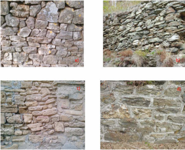
Figure 1. Irregular type of masonry a) b) d) Typical Lozerian structures, France c) Miramas-Le-Vieux, France.
