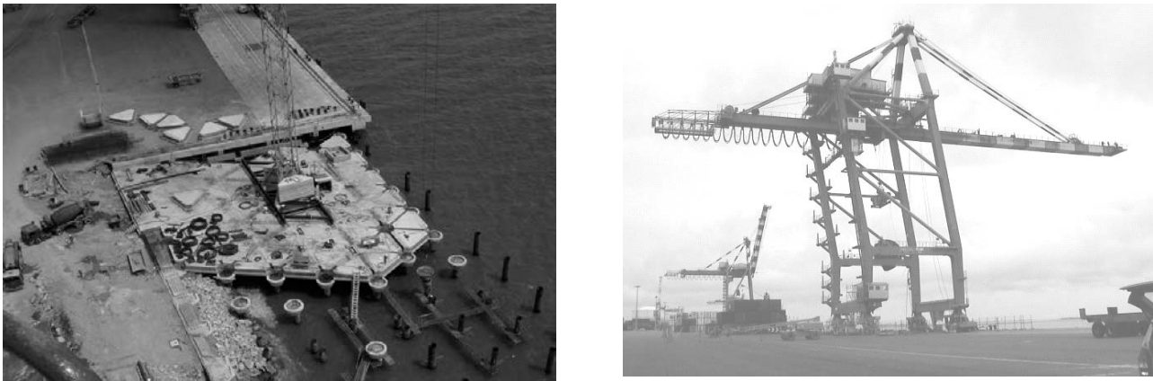
Figure 1. Aerial view of the wharf and a picture of the crane
