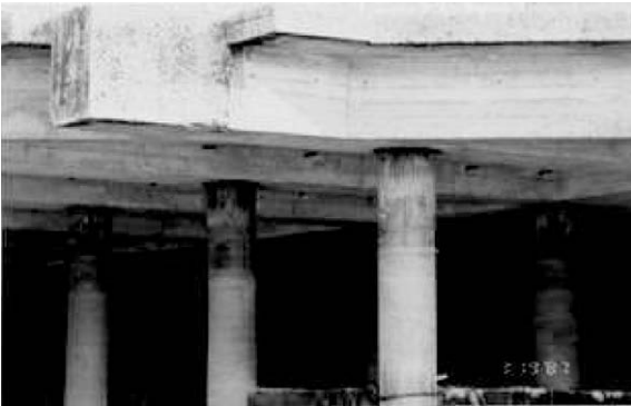
Fig. 6. Steel piles with corrosion.
