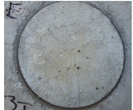
Figure 3. Test specimen face after one-hour exposure to propane flame
