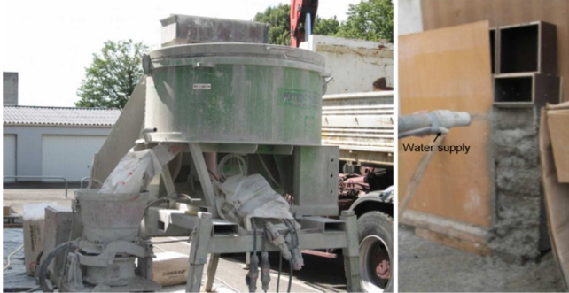
Figure 1. Spraying method (left : mixer, right : spraying hose)
