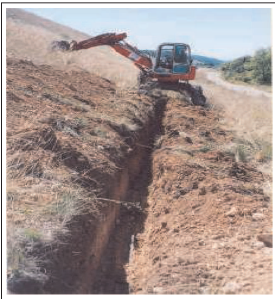
Figure 5. Digging up of the trench for optical fiber installation along the dike.
