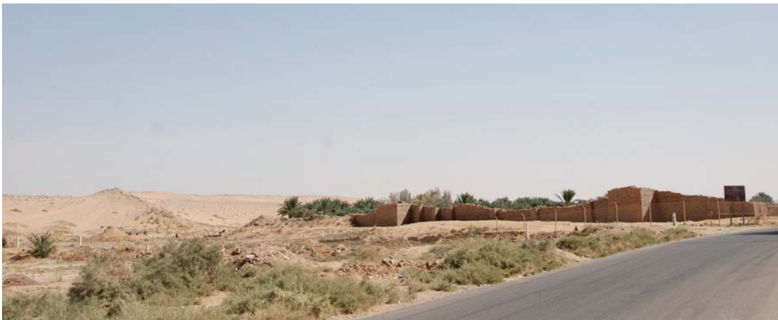
Fig. 14. Western wall unit 3, looking east
