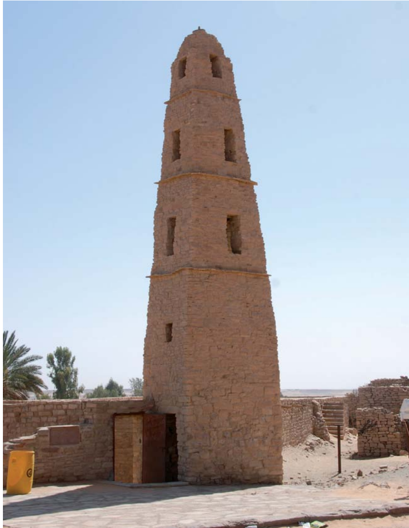
Fig. 12. The minaret of the ‘Umar bin al-Khattâb mosque
