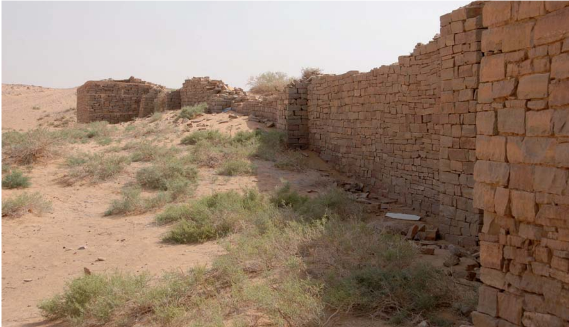
Fig. 75. Western face of the enclosure wall segment (unit 3) excavated in 1986, before cleaning, looking north
