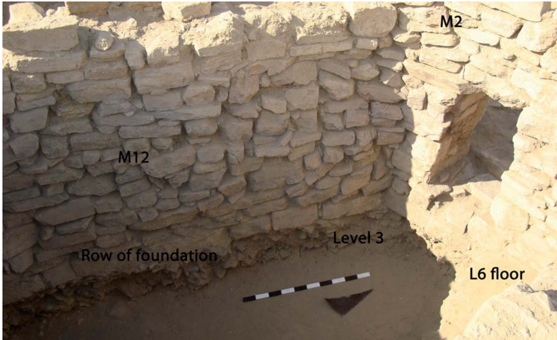
Fig. 26. L6 seen from inside. Its foundation courses are laid on a level of gravel (Level 3b)
