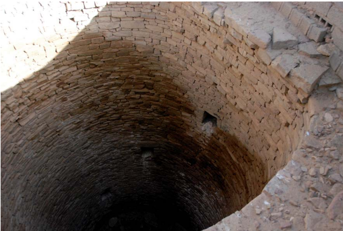
Fig. 14. Openings in the interior masonry of well PU1, near Qasr Mârid, looking north-west
