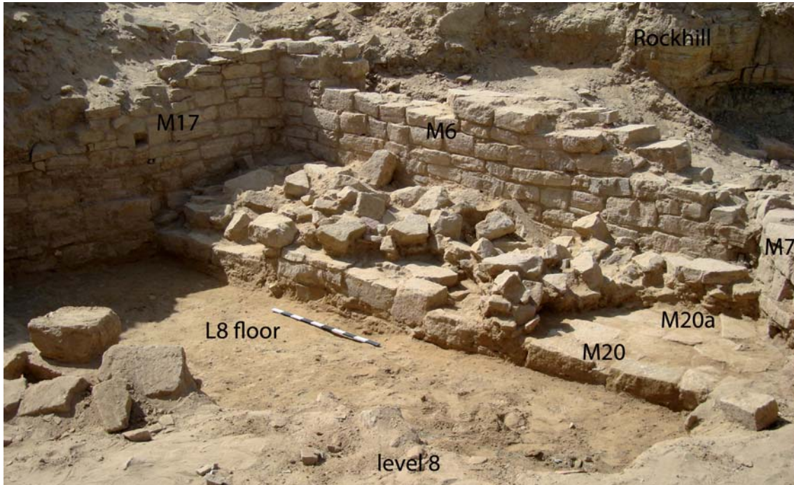
Fig. 48. Removal of the Middle Islamic structures made it possible to reach the structures relating to M6: M17, M20 pertaining to a building of impressive size and made using construction techniques which were more technologically advanced than the buildings in the medieval village
