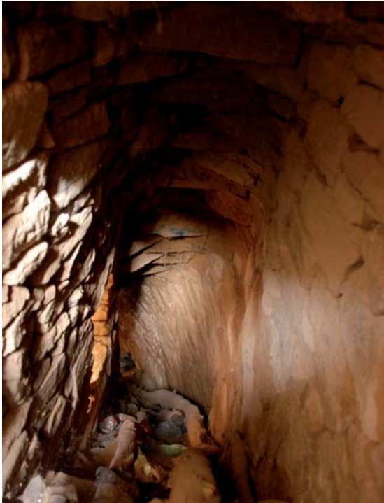
Fig. 15. Exterior staircae of well PU1, near Qasr Mârid, looking west
