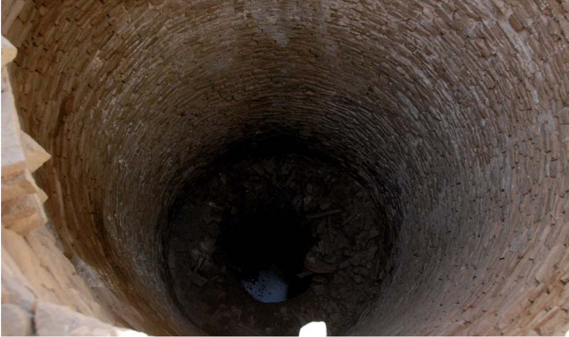
Fig. 13. Bottom of well PU1
