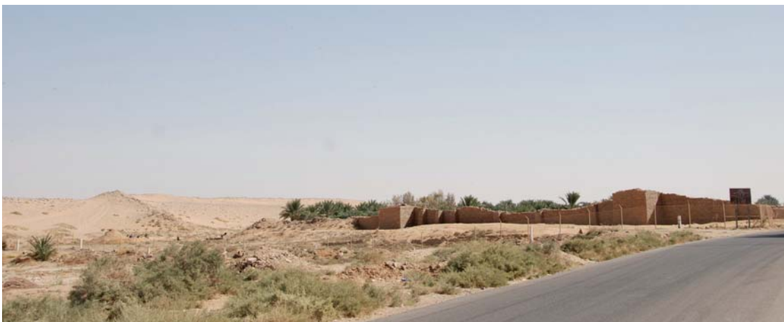
Fig. 14. Western wall unit 3, looking east
