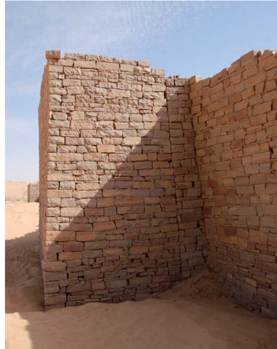
Fig. 19. Architectural cut between a stronghold and the western enclosure wall unit 3
