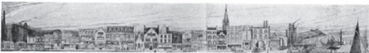
Starting from the left, the iron works and the shops of the ironmonger and goldsmith (miner) appear on the city street; then (woodman) timber and fuel yard, furniture shop, paper warehouse. Next the big (caravaneers') store with furs from hunter and woolen goods from shepherd. Also there is his small church or chapel with which there should be a school. The Hiring Fair, the original of the Labour Exchange, indicates the older appearance of the poor peasant, and in later times we see his bank and insurance company. The farmer occupies the street as miller, baker, brewer, butcher, greengrocer, innkeeper, etc. For the fisher is the fish shop and for the sailor and merchant venturer the warehouse and shipbuilding yard and the great seaports.
