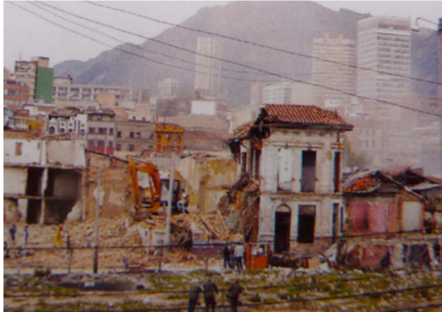
Demolition of Cartucho – Copyright reserved – Source Internet
