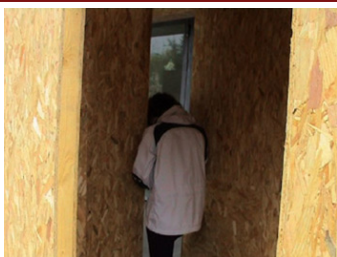
An original use of the telephone, ears are located between the two walls.
