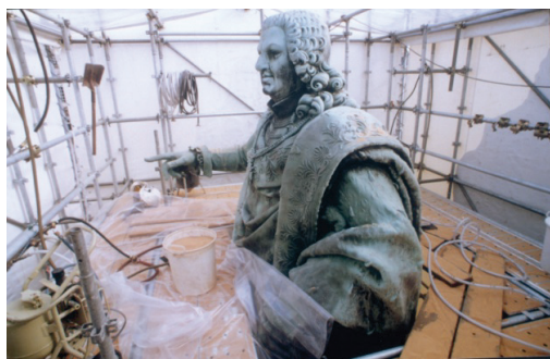
Figure 4. Cleaning of a bronze statue by walnuts shells with an air abrasive technique.
